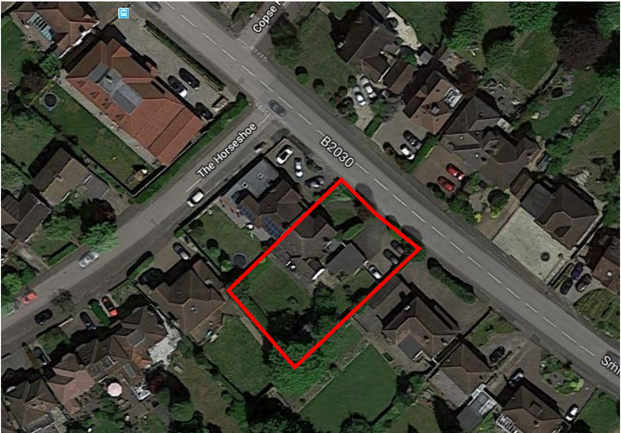
Fig 1: Aerial street view highlighting the proposed site within the surrounding streetscene
